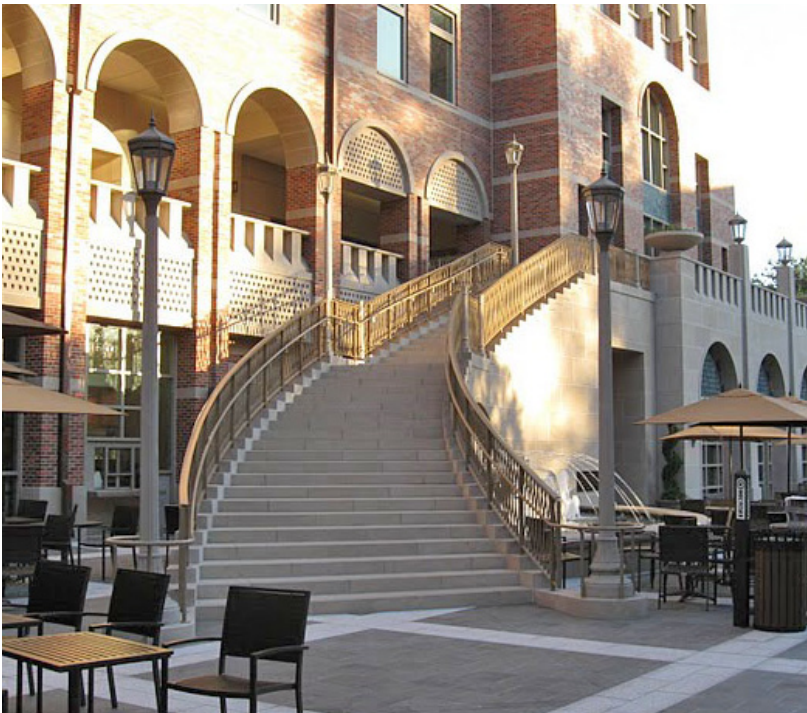
Stair trades were made using architectural precast. Each trade had a unique shape, size, and curve. The AAS team used different molds for each of these trades. The balustrades in the building have a unique design. They were made using cast stone.
