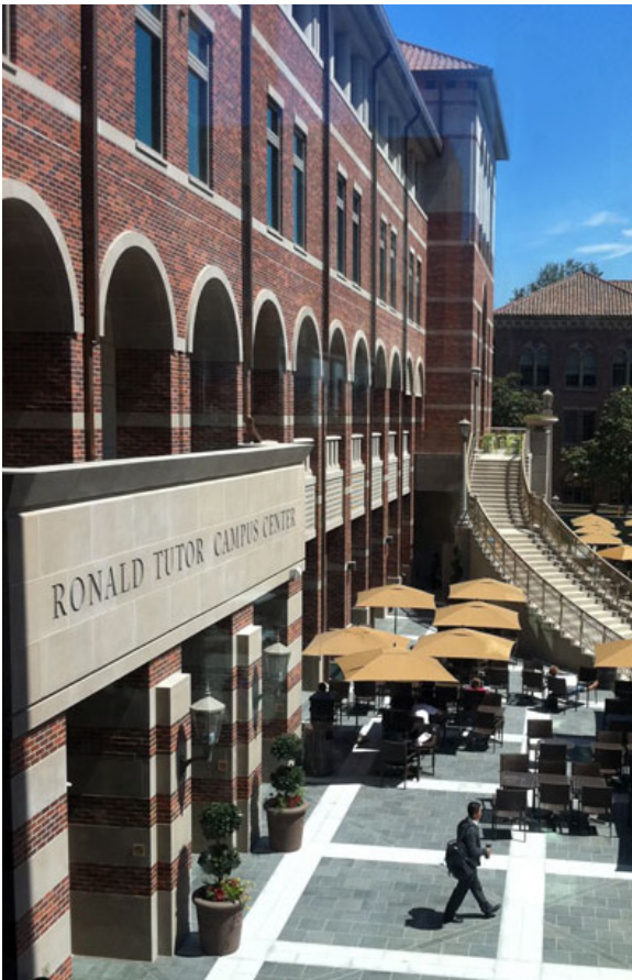
Precast was used heavily in the design of the structure – from the base of the buildings, to stairways, terraces and garden ornamentation.
