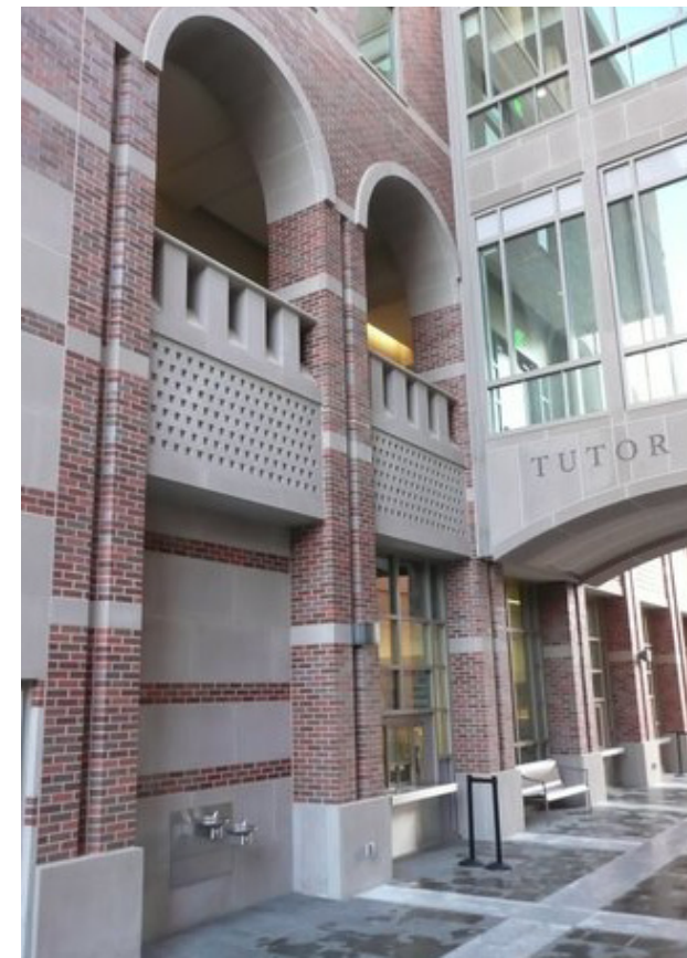
The columns at the high elevation used GFRC for light weight.
