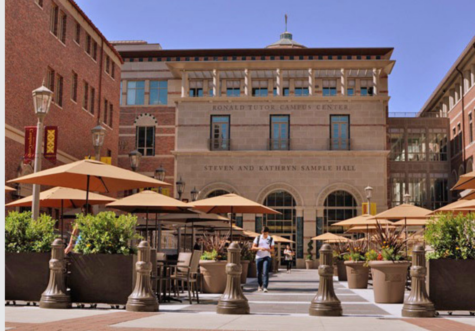
The columns at the high elevation used GFRC for light weight.
